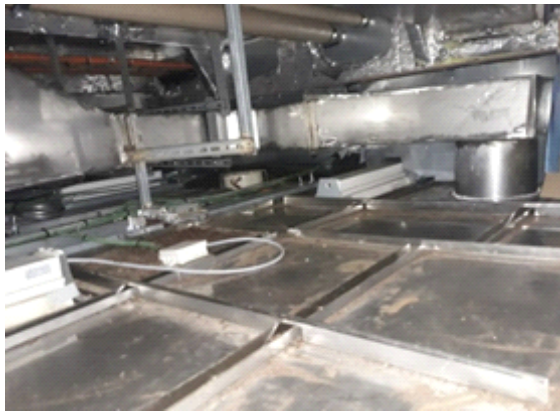
Galley ducts replacement
