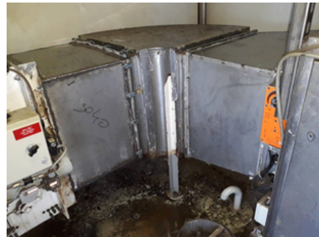
Repair of inlet duct – after
