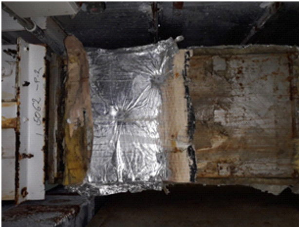
Repair of inlet duct – before
