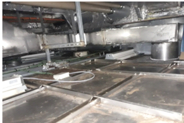
Galley ducts replacement
