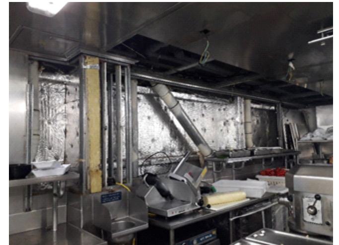
Dismounting of galley walls and ceilings
