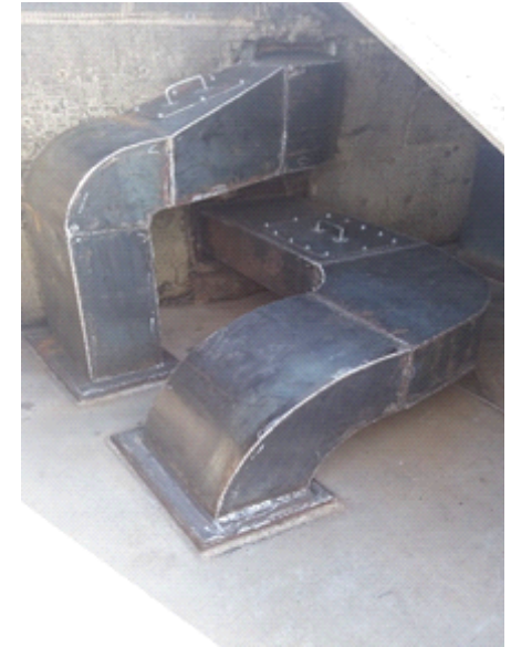
Inlet ducts after
