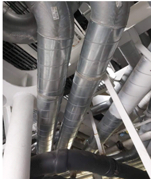
Circular ducts replacement
