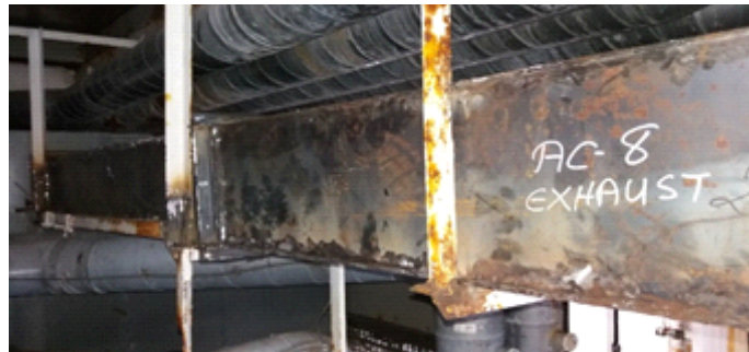
Exhasut duct replacement
