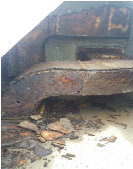
Inlet ducts before
