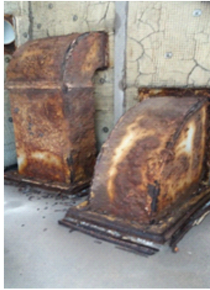
Inlet ducts before
