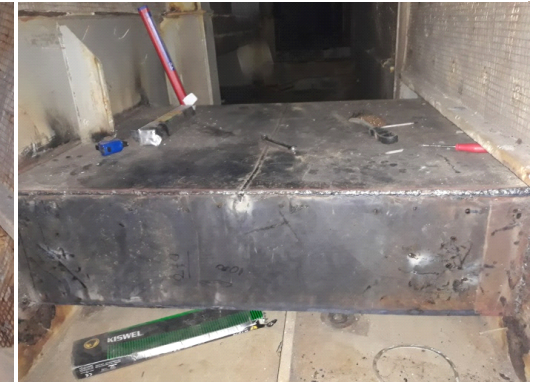
Inlet duct after
