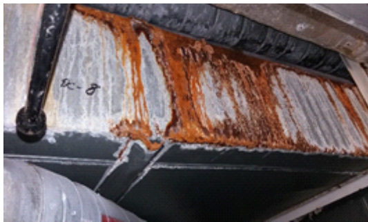
Exhasut duct replacement
