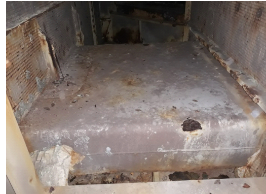
Inlet duct before
